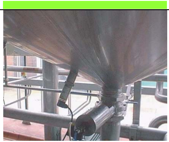
Figure 2: The compact vibrating fork level switch is easily mounted in bottom of the tank. The short fork ensures minimum intrusion.
